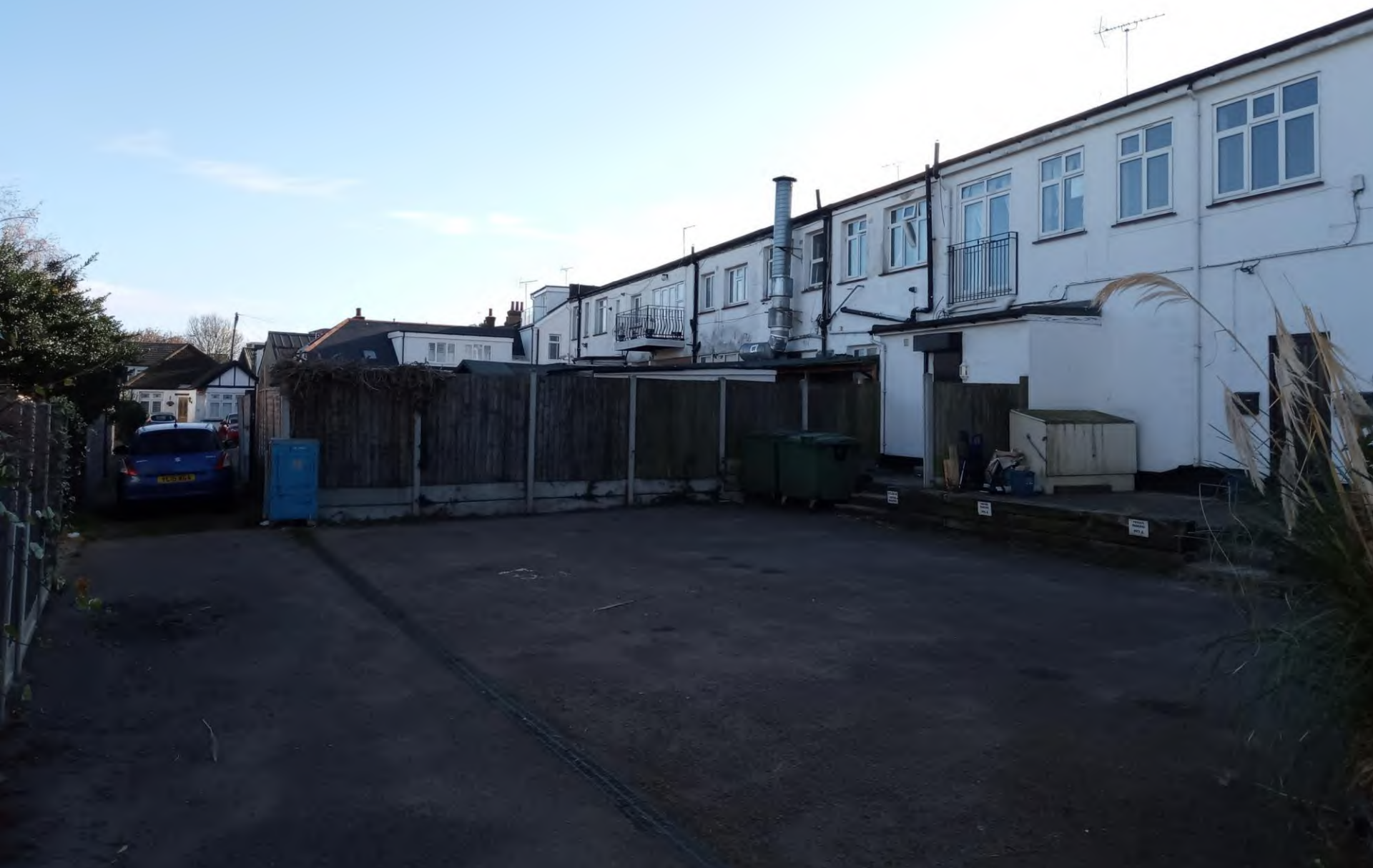
Rear of site
